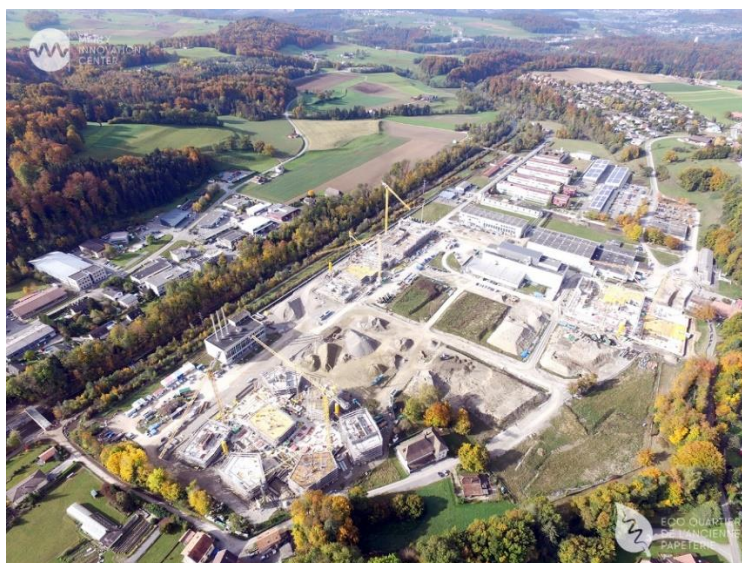
Figure 1 - Marly Innovation Center – Chantier Ecoquartier 2021
